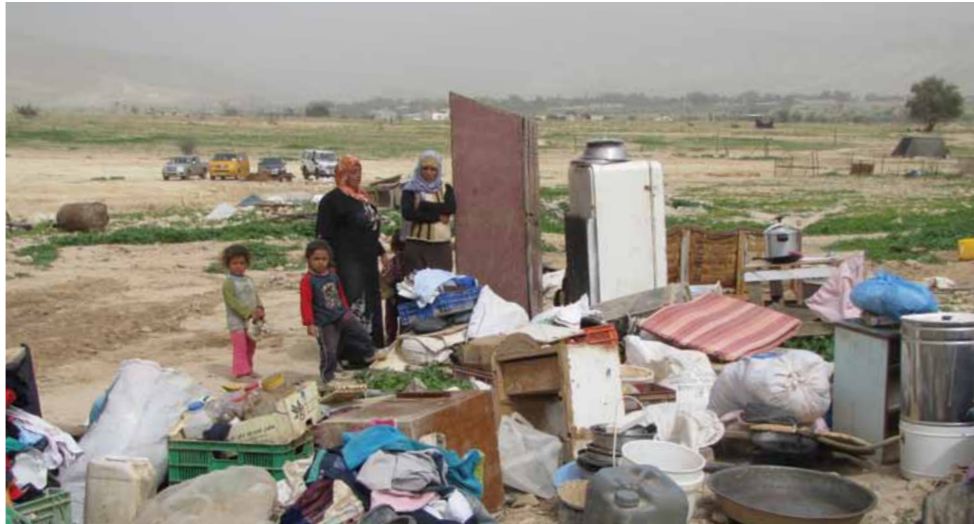
▲ Members of the a-Rashaydah family after the demolition of their home in Fasayil, the Jordan Valley. Photo: B'Tselem/Atef Abu a Rob
