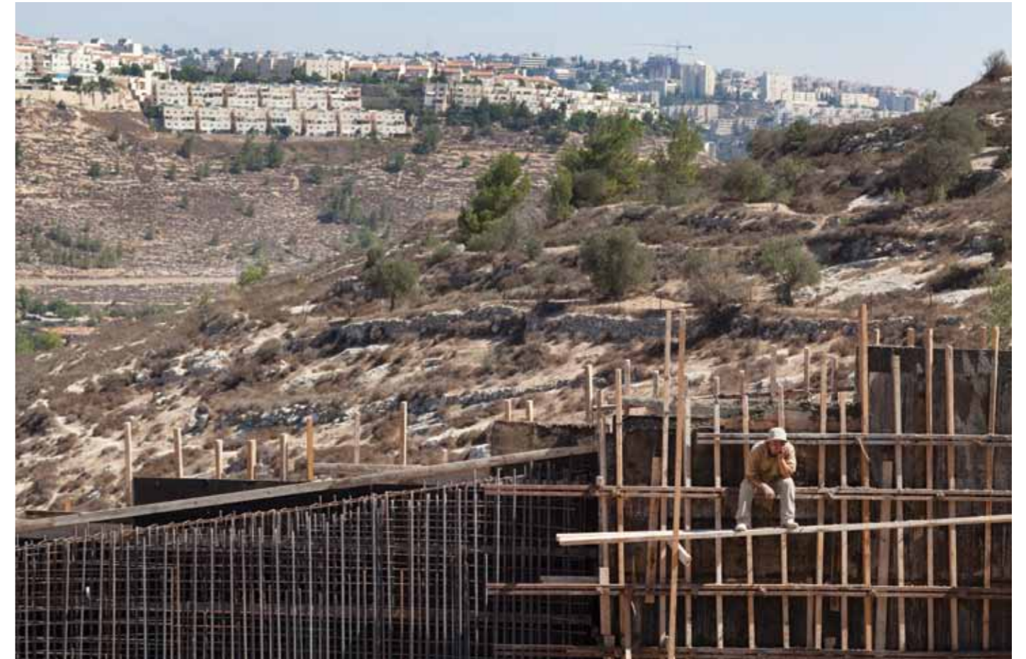
▲ The construction of the Wall in the Palestinian village of Al Walaje which has been surrounded by thousands of settlement units in the Gush Etzion bloc. Photo: David Levene
